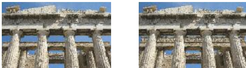
The west façade of the Parthenon during the intervention and after completion of the restoration.
