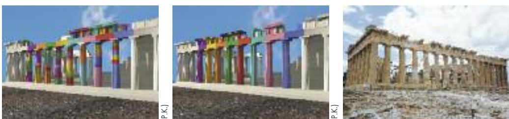
Digital imaging of the north colonnade, with different colours indicating the misplaced drums before the restoration, and after repositioning in their original places.
