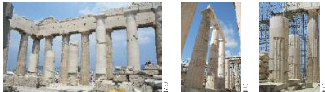
The pronaos of the Parthenon during the restoration.
